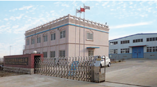
Qingdao Office & Factory China
